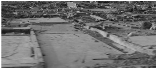
Fig.1 A photograph of a Miyazaki City after Tsunami attack. Almost all building had lost
